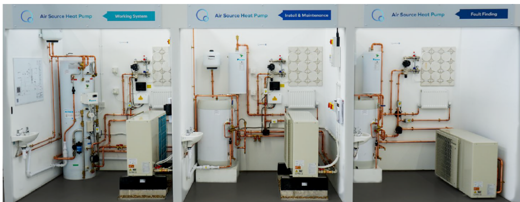
Air source heat pump bays
